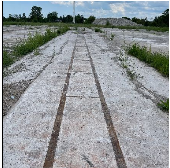
Image 4 : Area of disturbance former factory.
