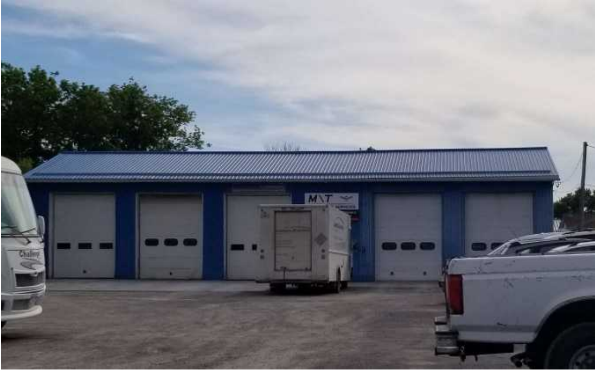
Photo 11: M/T automotive services which operates as a automotive repair and maintenance facility (PCA 10) at 31 Tripp Avenue
