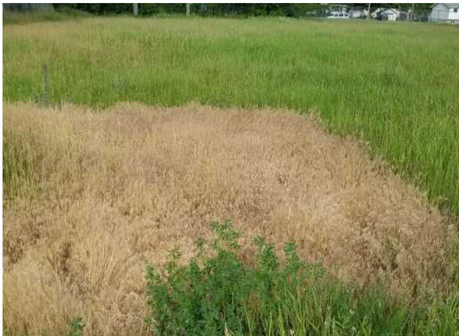
Photo 4: Distressed vegetation associated with the buried UST just south of the tank
