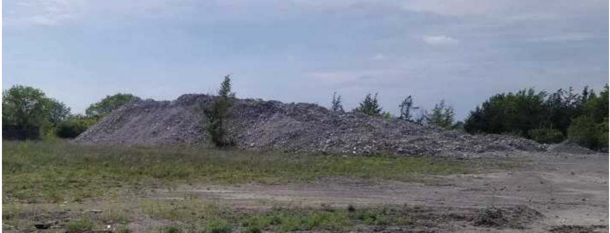
Photo 15: Large material (fill) pile (PCA 30) consisting mostly of concrete located near the north property line of the Phase One Property (western portion) looking towards the northwest
