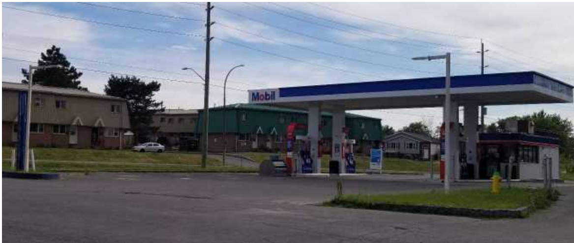
Photo 10: Mobil gas station at 269 Moira Street West ventilation pipes for four USTs observed on the left
