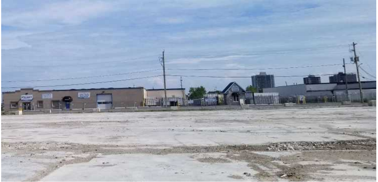
Photo 1: Eastern portion of Phase One Property looking towards south at the foundation of main building and Wilson Ave
