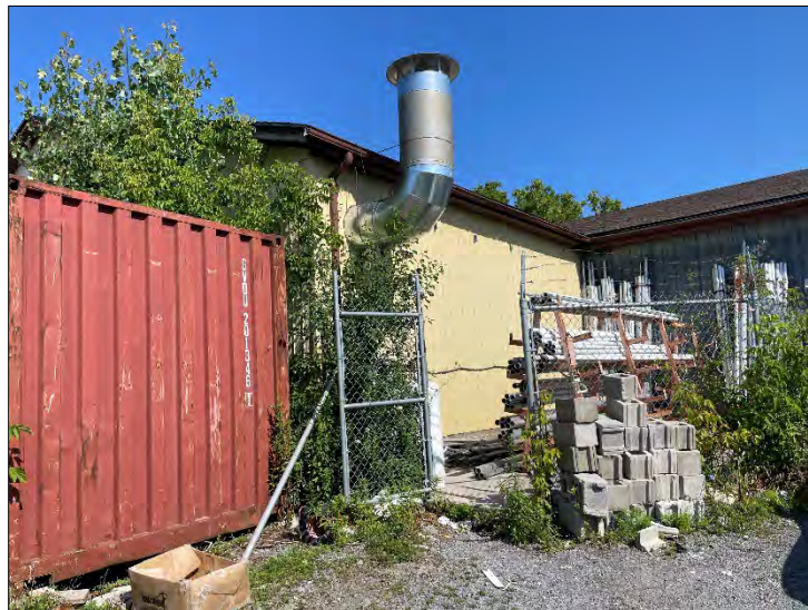
Side View of 84 Cannifton Road N main building. Picture is taken facing northwest.
