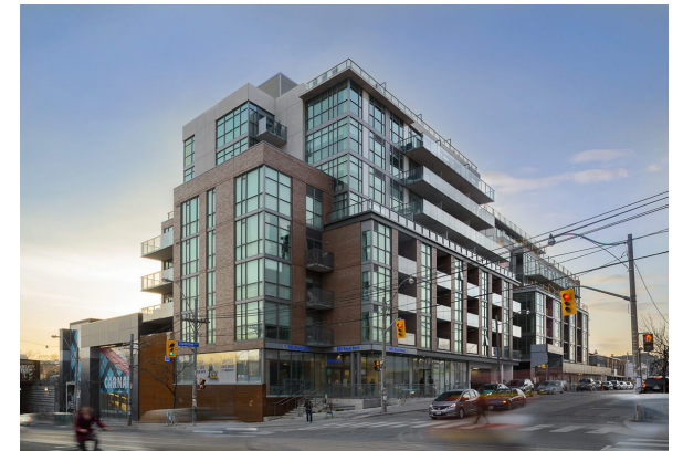
8-storey Mixed-Use Residential (Toronto, ON)
