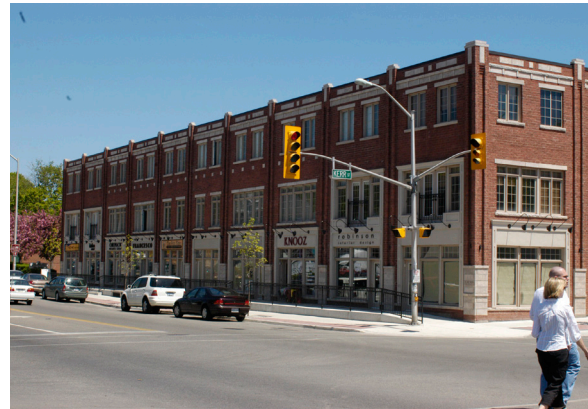
3-storey Mixed-Use Residential (Mississauga, ON)
