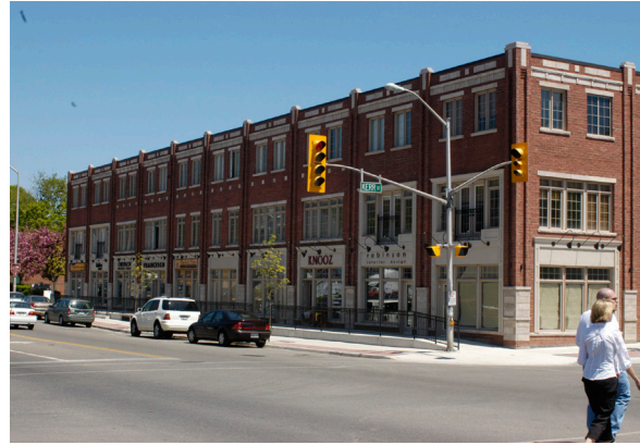
3-storey Mixed-Use Residential (Mississauga, ON)
