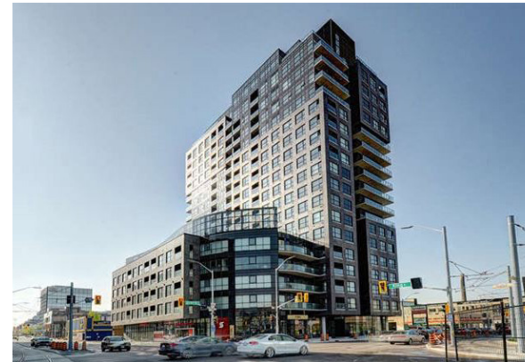
Slab/Podium Mixed-Use Residential (Kitchener, ON)
