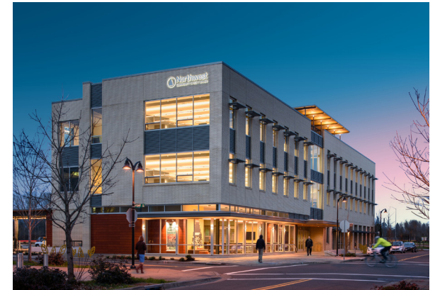
3-storey Mixed-Use Office (Portland, OR)
