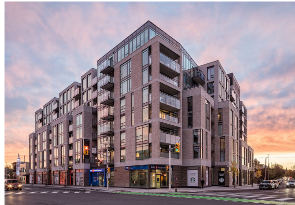
8-storey Mixed-Use Residential (Mississauga, ON)
