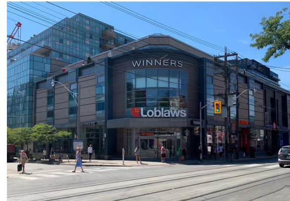
4-storey Mixed-Use Commercial (Toronto, ON)
